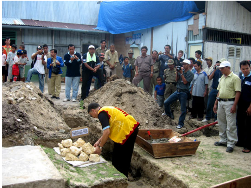
Laying the stone to mark the start of housing construction process
