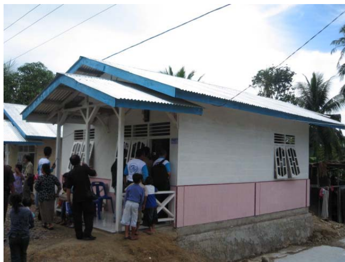
UN-Habitat's house in Hilimbosi village, Tuhemberua sub-district, Nias (Photo: UNORC Nias)
